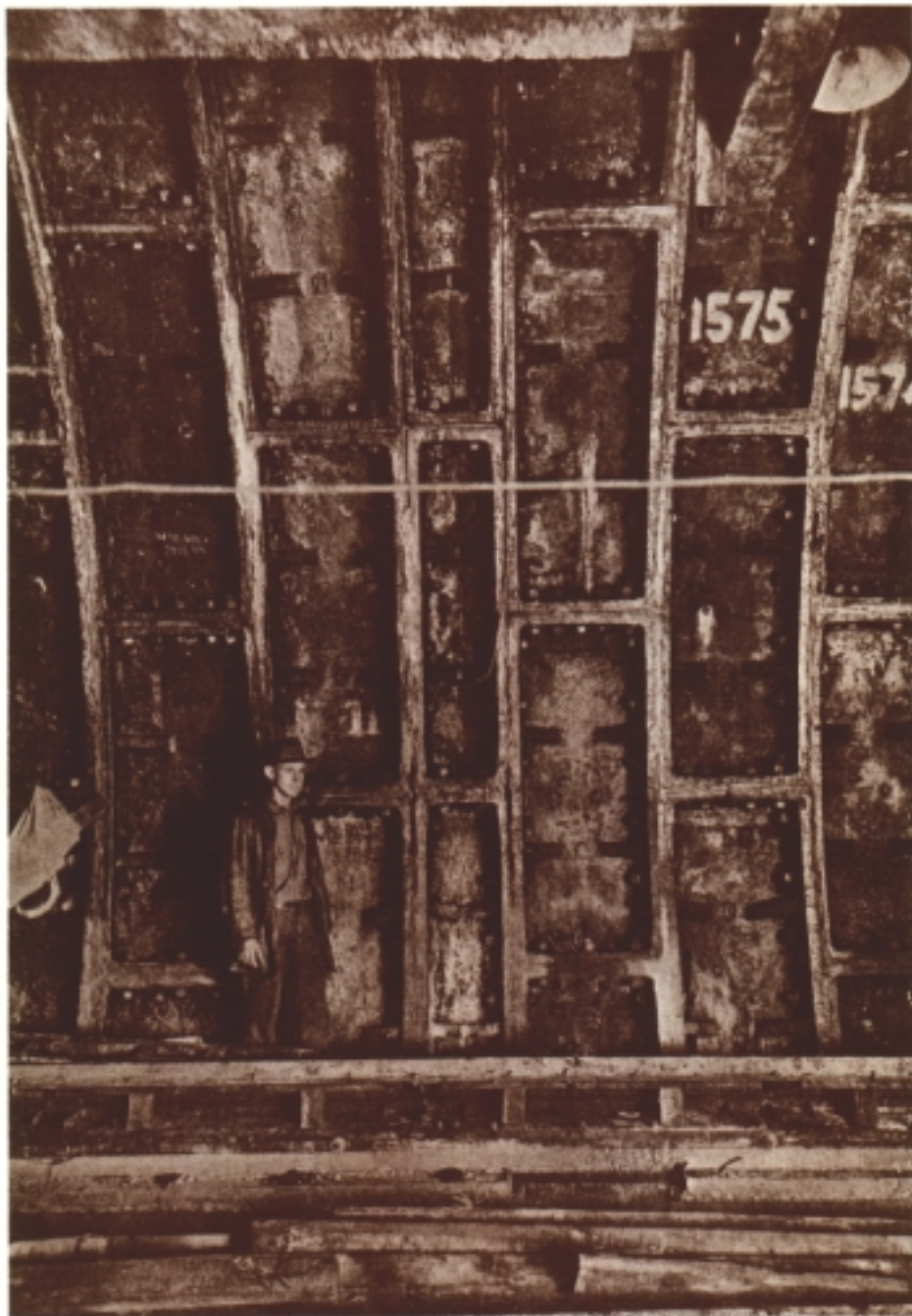
CLOSER RING AT JUNCTION OF SHIELDS, NORTH TUNNEL.
