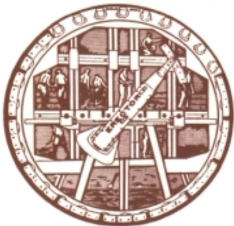
REAR OF SHIELD- ERECTION OF CAST IRON TUNNEL RINGS
