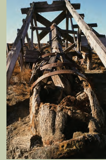
BASE OF OLD PUMP SHOWING REMAINS OF HELIX.
