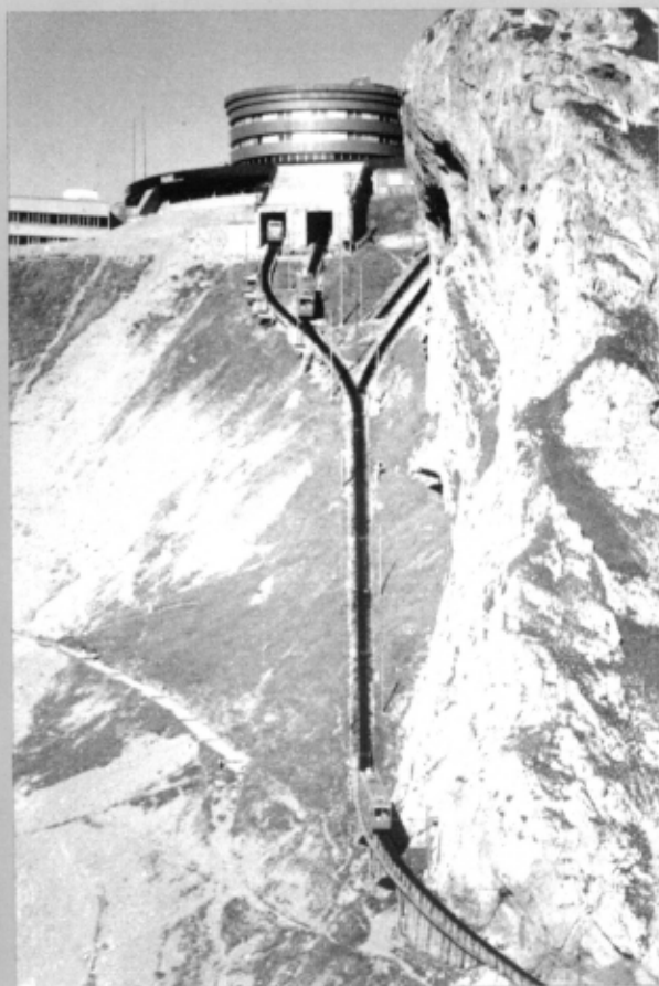
(bottom right) This overview of the mountain station shows limitations posed by the terrain and the need for a unique design for the track switches, or turnouts.
