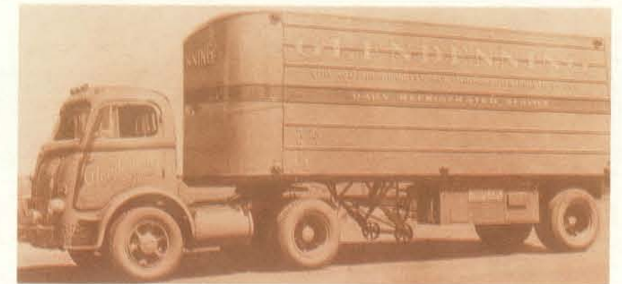
Mounted underneath the trailer, the Thermo King Model A was the first workable, mechanical transport refrigeration system.
